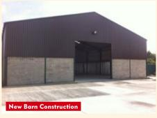
▲ Construction of a steel portal framed agricultural building with profiled steel cladding to roof and walls at high level
